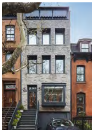
33 106 Prospect Place, Brooklyn Architect: James Cleary Architecture Completed: 2016 Brick: D91 DNF Photo: Dean Kaufman See article on page 9
