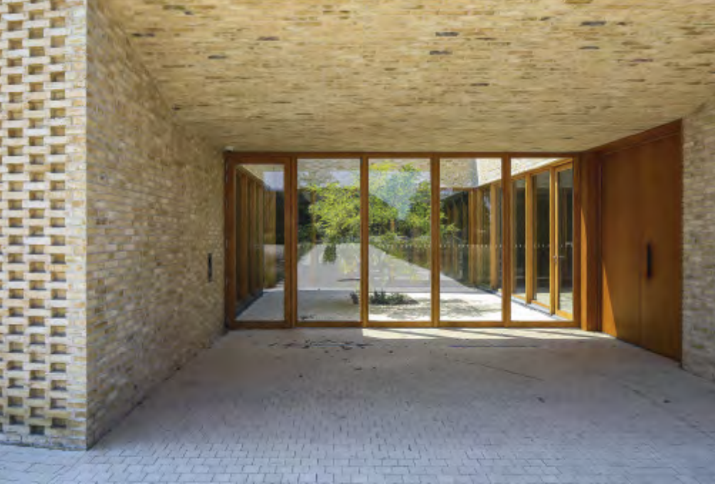
The main entrance seems to have been cut into the body of the building. Even the sloping ceiling is in brick, adding to the sense of mass of the building as a whole. An atrium draws light into the centre and serves as a place to take breaks. Photo: Paul Kozlowski
