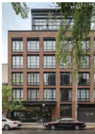
15 438 East 12th Street, Manhattan Architect: S9 Architecture Completed: 2017 Brick: D43, D37, D54 DNF Photo: Florian Holzherr See article on page 6
