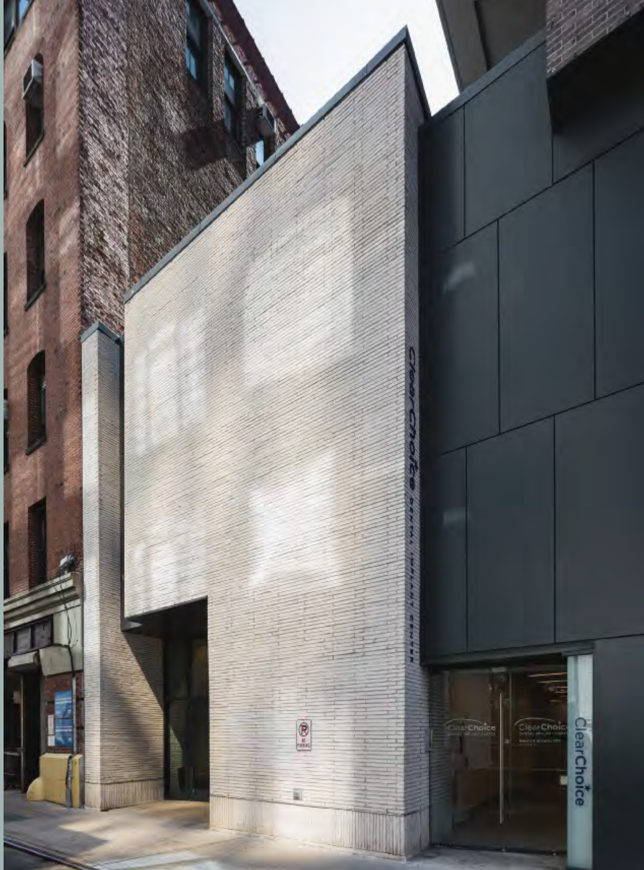
The tall residential block and the sharply defined entrance building are visually separated by a black-painted steel section. For the entrance, the architects chose the almost white K11 brickwork in a quarter-brick block bond. The bond stands out due to the colour of the joint, which is slightly darker than the brick. At ground level, the building has a course of headers.
